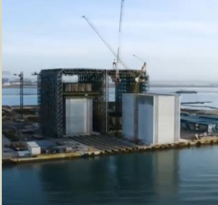
CAISSON READY FOR LAUNCHING
