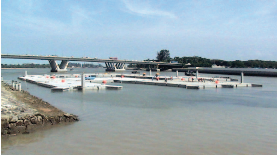
Figure 16. Assembly of floating pontoons on-site
