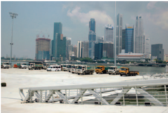
Figure 17. Load Testing of floating platform
